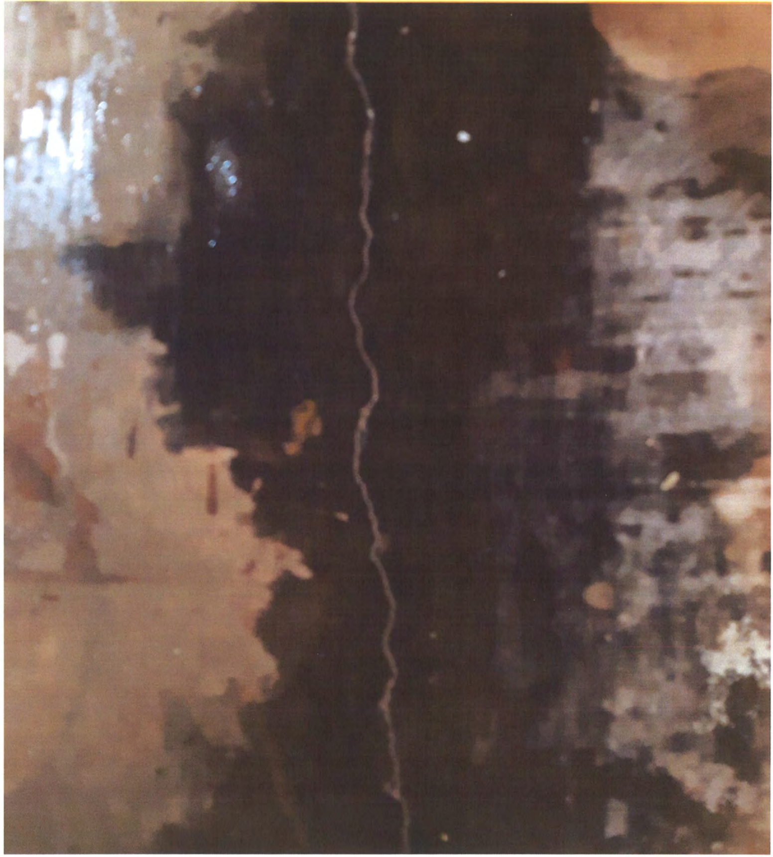
Crack in basement floor
