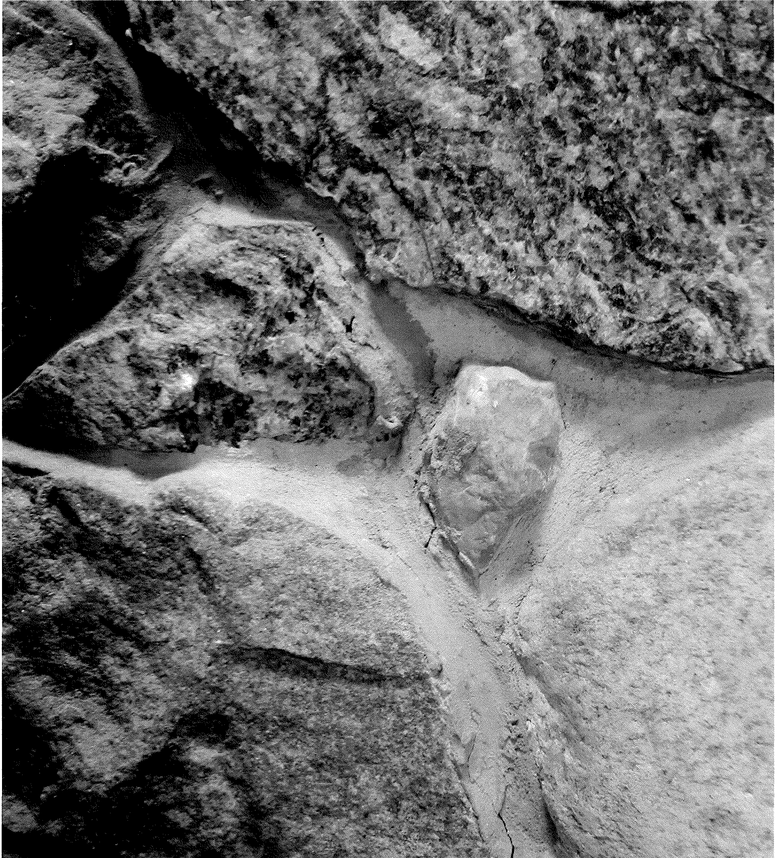
Crack in fireplace wall - Ms. Ladd tried filling cracks herself
