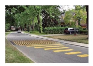
safety. Like speed humps, discomfort increases as the speed of the vehicle traveling over the hump increases. Speed tables are good for locations where low speeds are desired, but a somewhat smooth ride is needed for larger vehicles.
