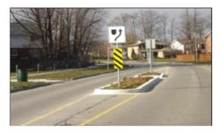
adequate travel lane width on either side of the median island to accommodate snow clearing efforts, as well as ensuring adequate sightlines can be maintained should vegetation be planted in the raised median. There are also ongoing operating costs associated with sustaining vegetation in the raised median islands.
