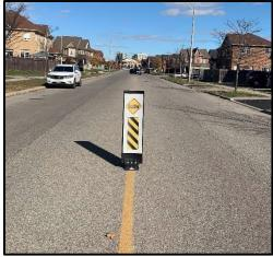
The signs do not represent a controlled crossing opportunity for pedestrians. The signs can be installed on local and collector roads with two-way traffic flow.
