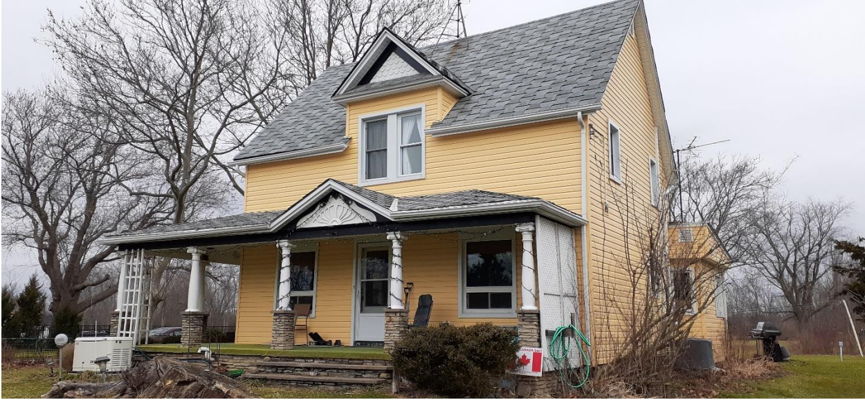
Fig. 11. Front (south) façade
