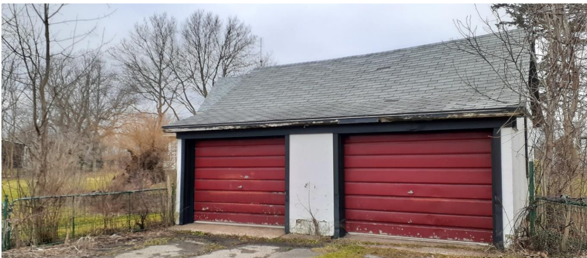
Fig. 1 Old Blacksmith Shop south side 5446 Sherkston Road facing Sherkston Road
