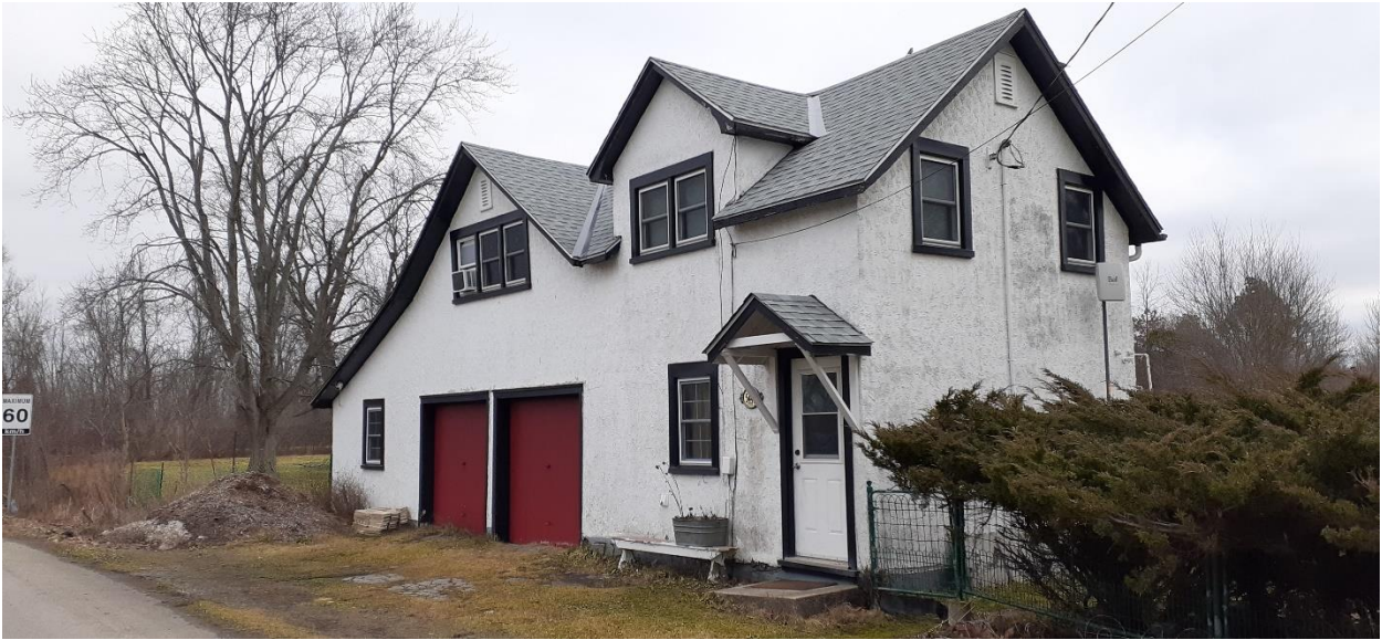
Fig. 6 Old stables west and south sides
