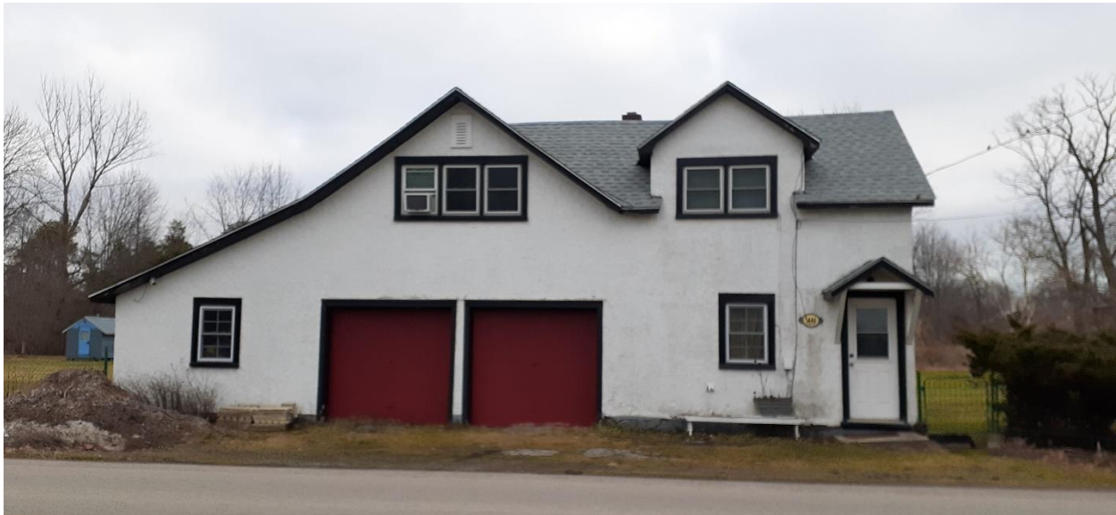
Fig. 5 Old stables facing Pleasant Beach Road west side
