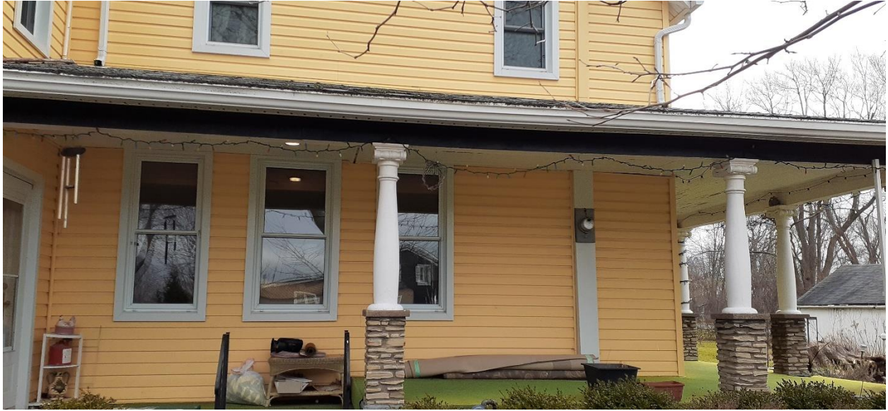
Fig. 13. Porch and west side, house at 5446 Sherkston Road/825 Pleasant Beach Road
