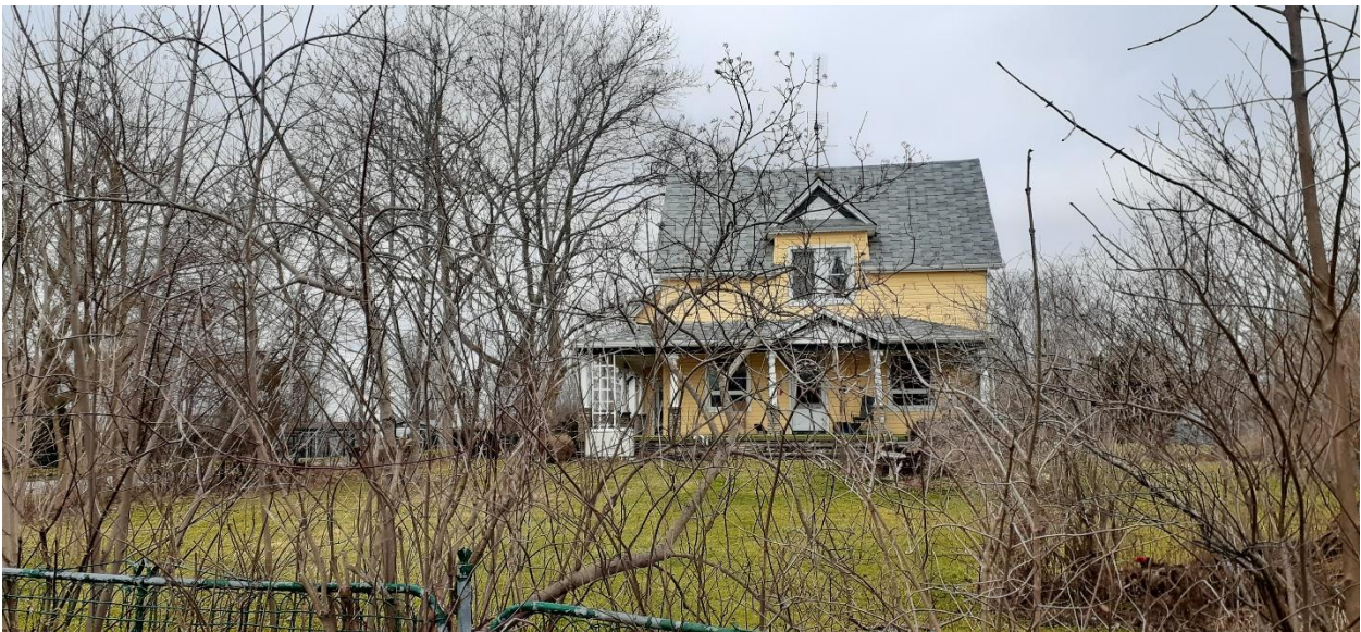
Fig. 10. House, 5446 Sherkston Road, south (front) façade facing Sherkston Road
