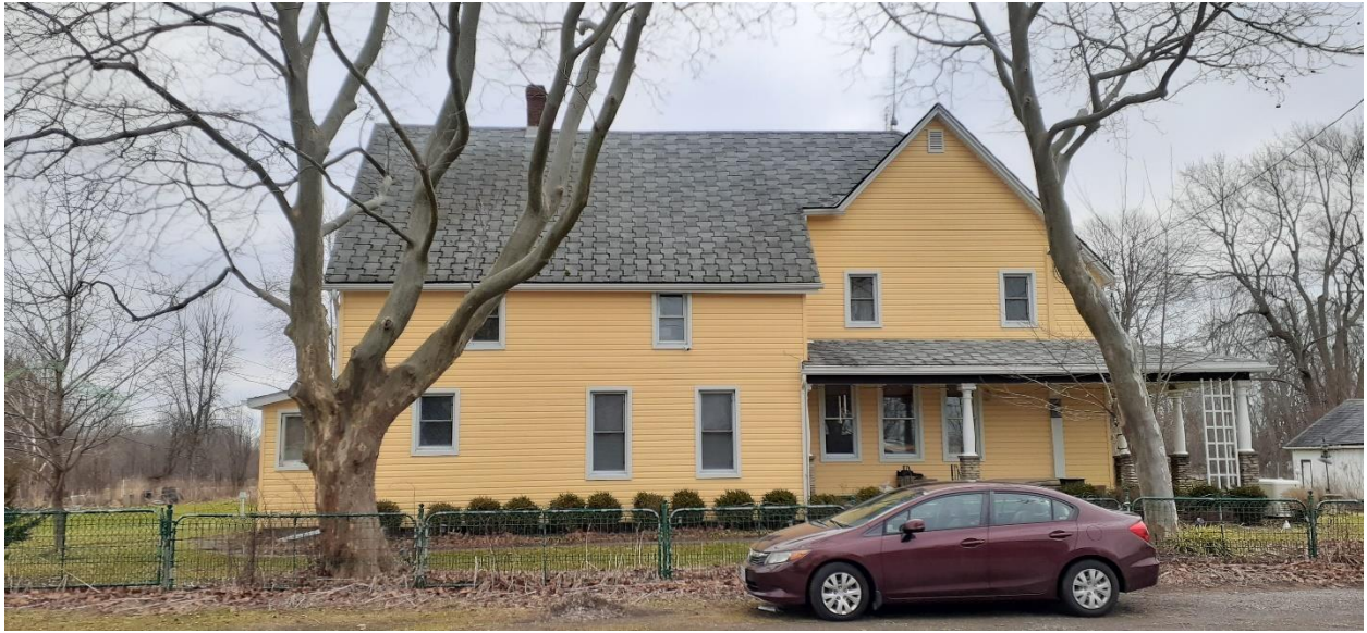
Fig. 14. Porch and west side, house at 5446 Sherkston Road/825 Pleasant Beach Road
