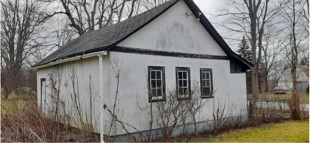
Fig. 2 Old Blacksmith Shop west side 5446 Sherkston Road
