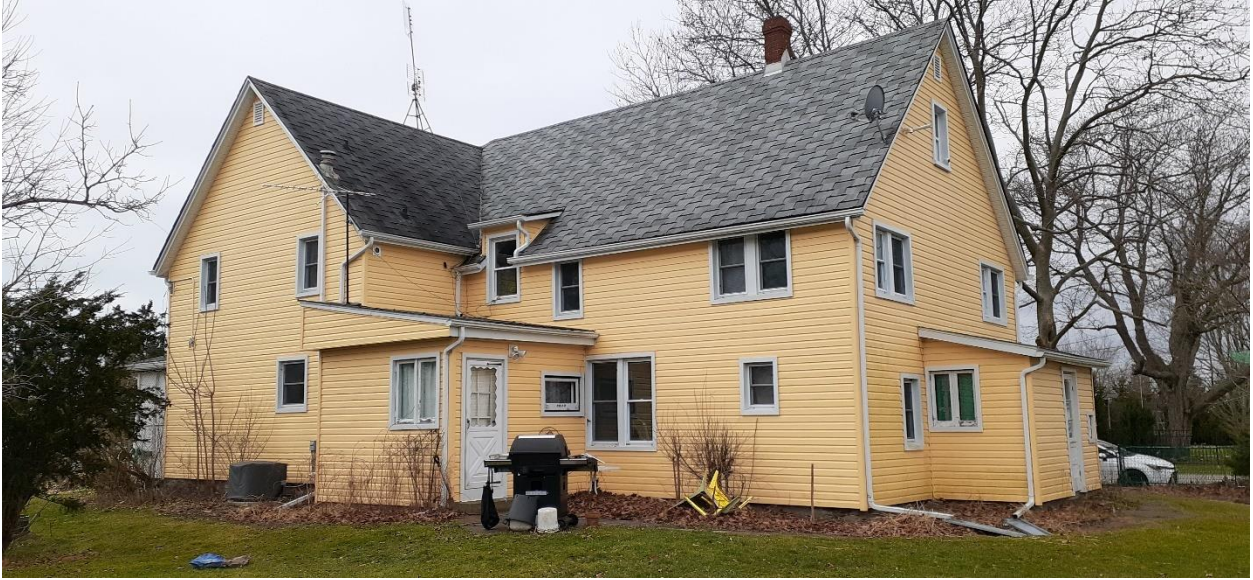
Fig. 16 East side of house, 5446 Sherkston Road
