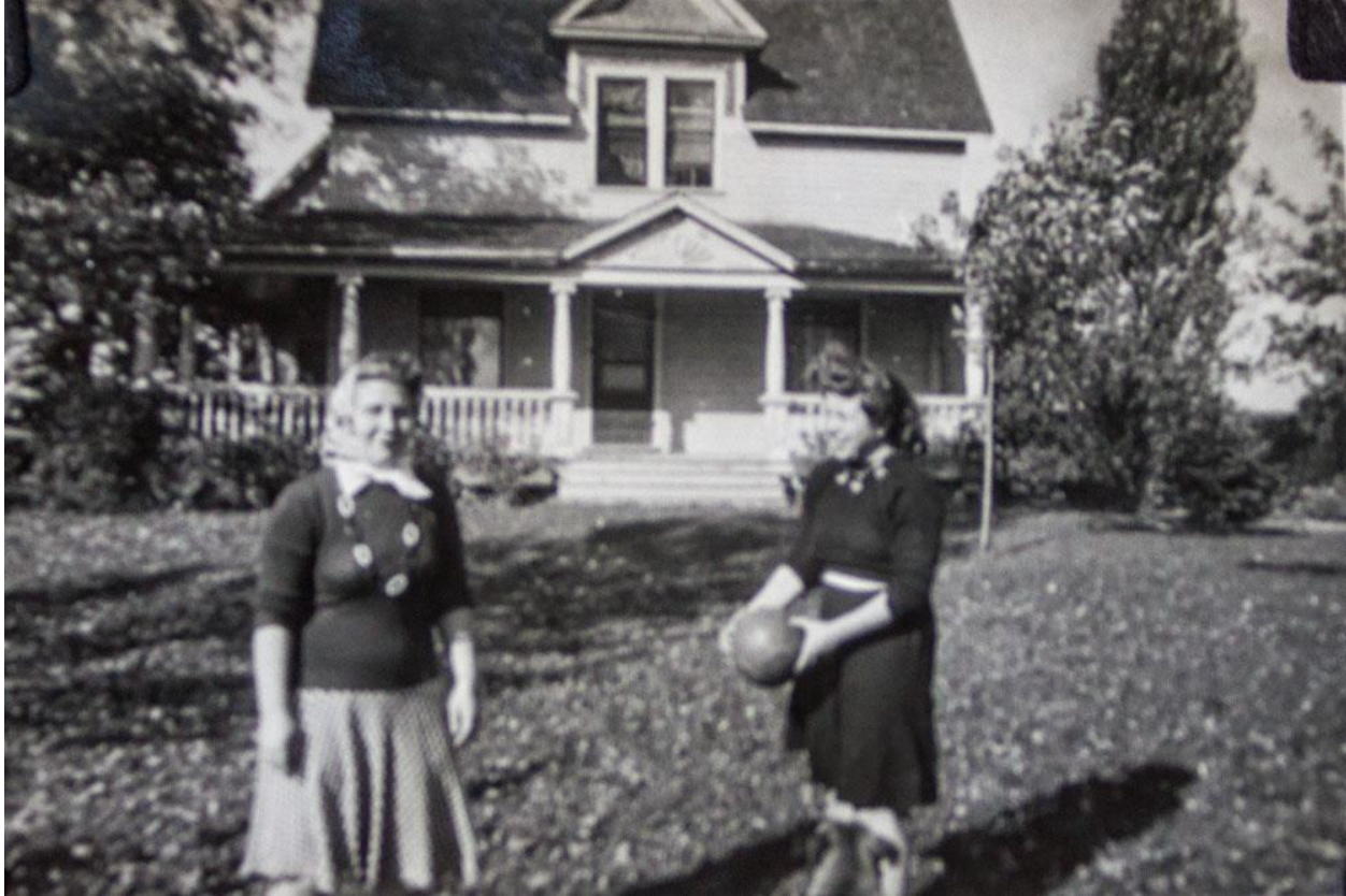
Fig. 20 Front façade of house c. 1930's
