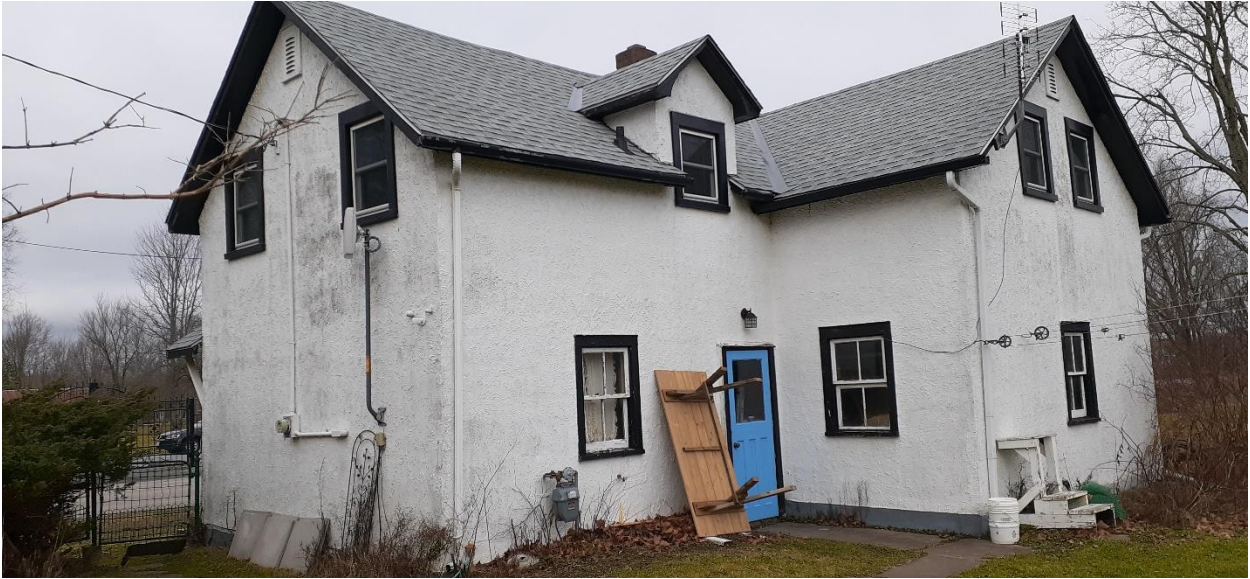
Fig. 7 Old stable south and east sides
