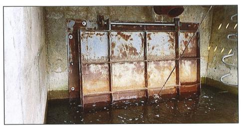
Figure 5 OMC Outlet Flap Gate
