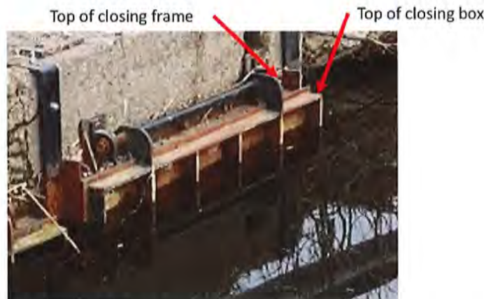
Figure 1 Existing gate after being rehung
