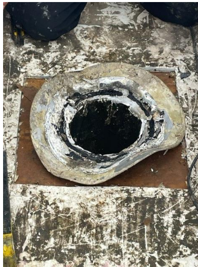
Existing drains in gutter (6-8" stack jacks)
