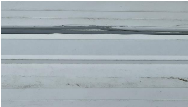
Typical damaged standing seam
