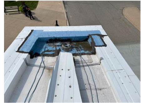
Existing Gutter Temporary Repair
