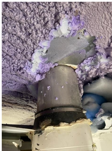
Existing 2lb insulation 1.5" thick (R9) (Interior)
