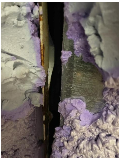
Air gap between gutter pan and insulation
