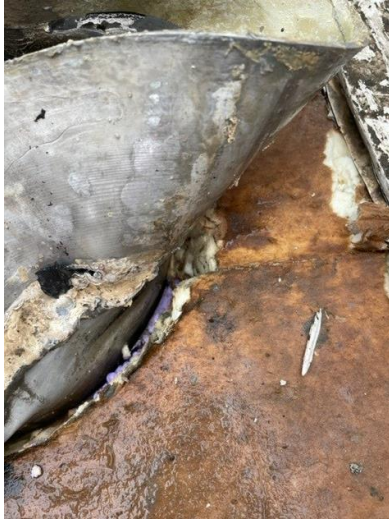
Existing drains in gutter (6-8" stack jacks)
