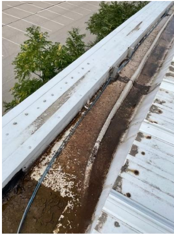
Creased South Gutter Liner
