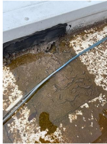
Failing Gutter Liner Patches
