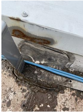
Failing Gutter Liner Patches
