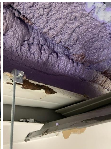
Insulation required on back side of C channel (Interior)
