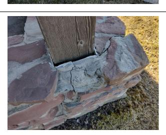
The wood column at the northwest corner is deteriorated where visible within the stone base. There is also notable movement of the column. The column is not supported.
