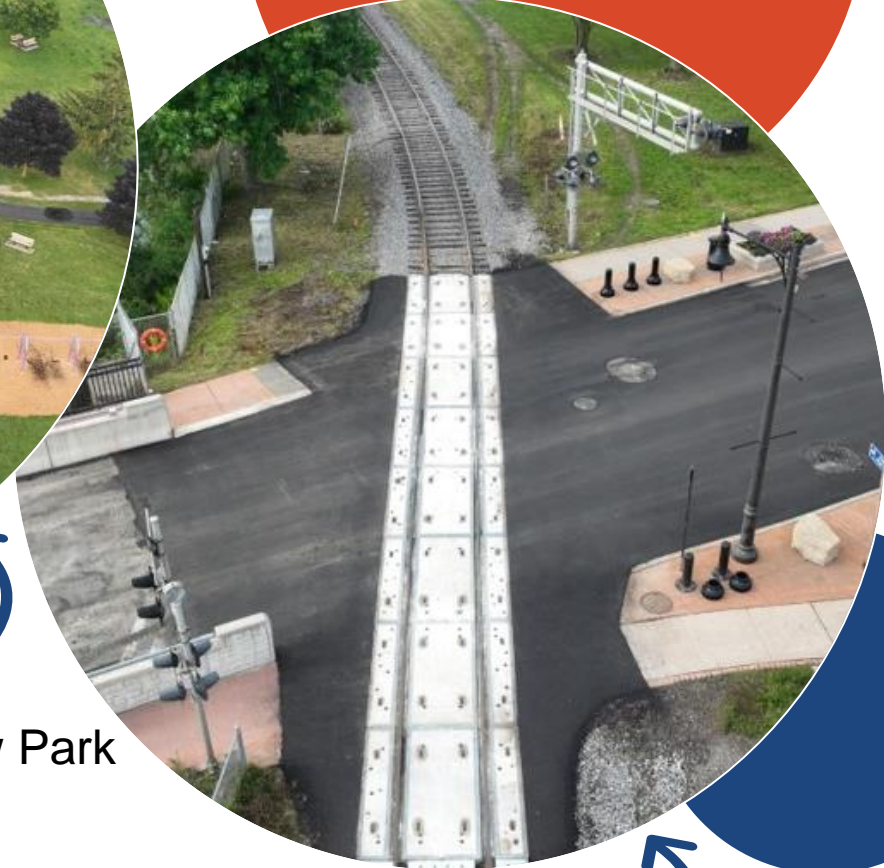
Main St Rehabilitation
