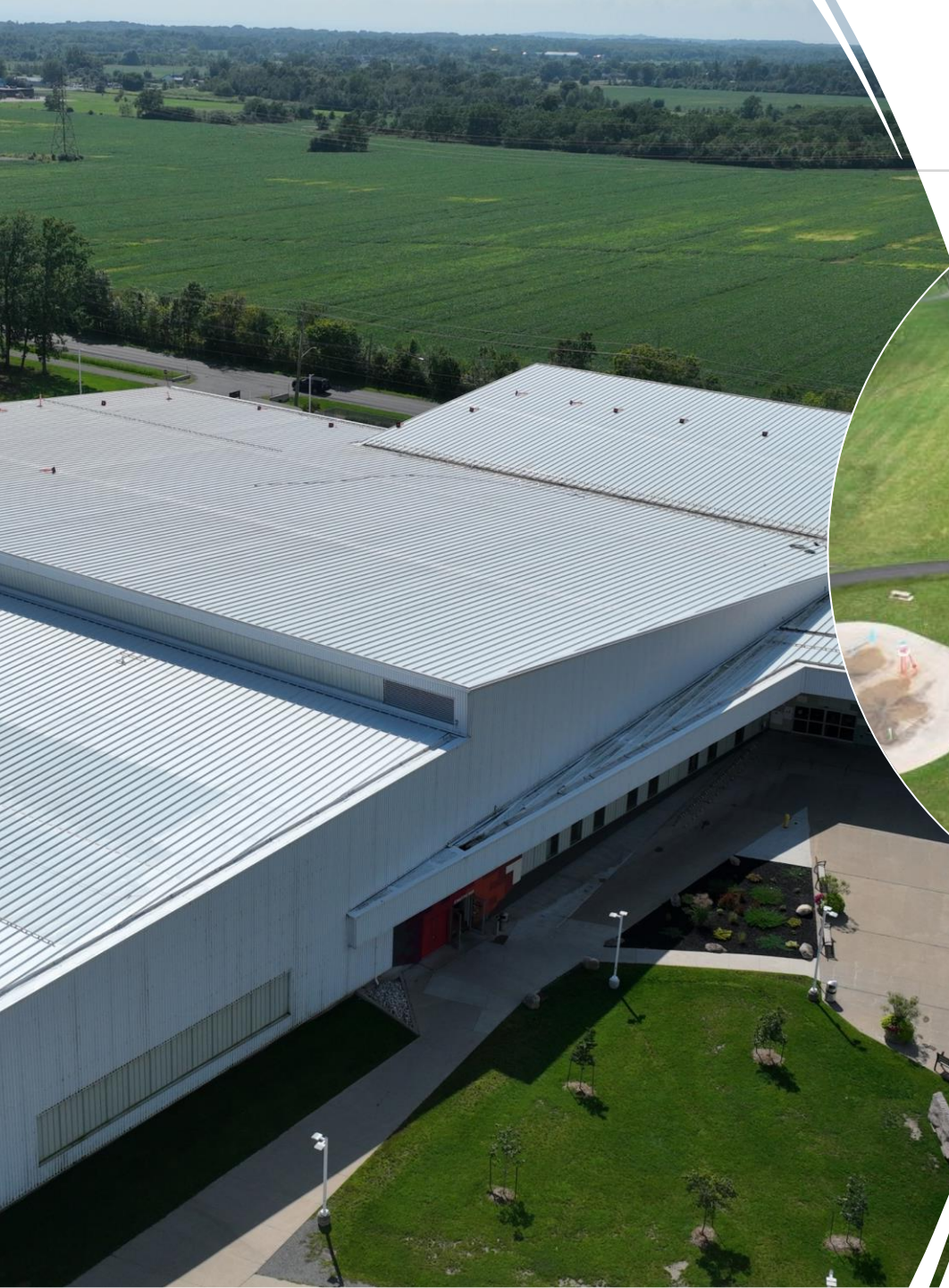
Vale Health & Wellness Centre roofing project
